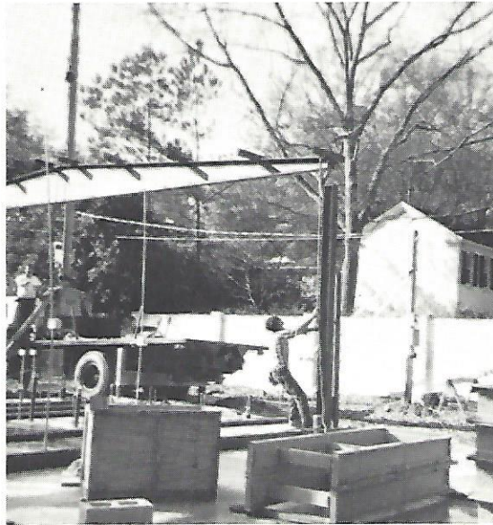
then you put up the steel posts
