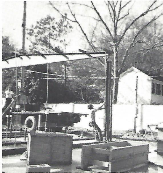
then you put up the steel posts
