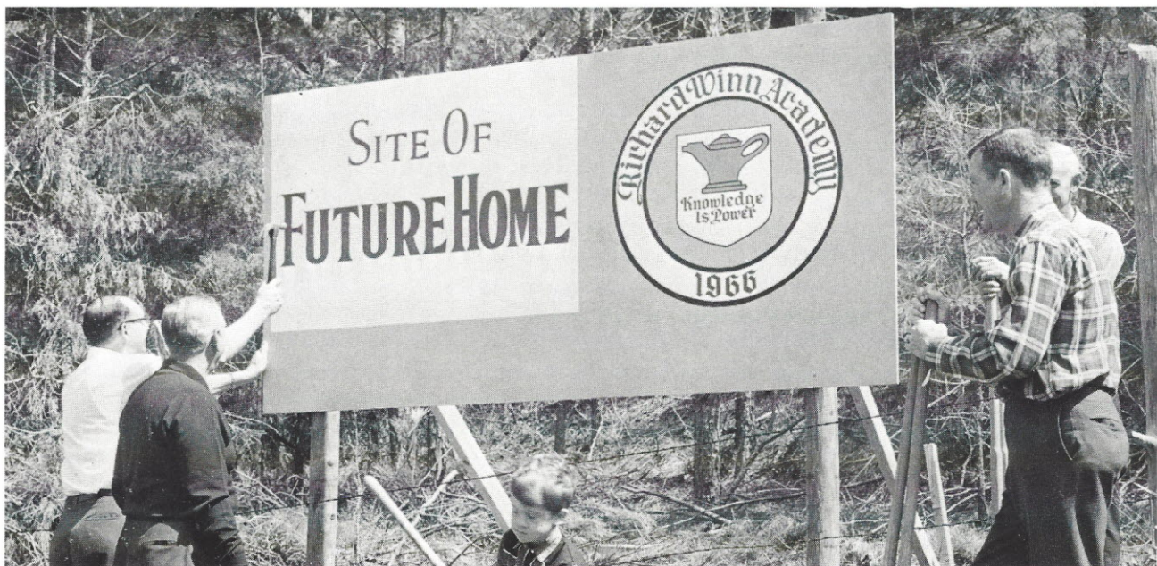
Some of the directors erecting a sign on the site of the future home of the Academy.
