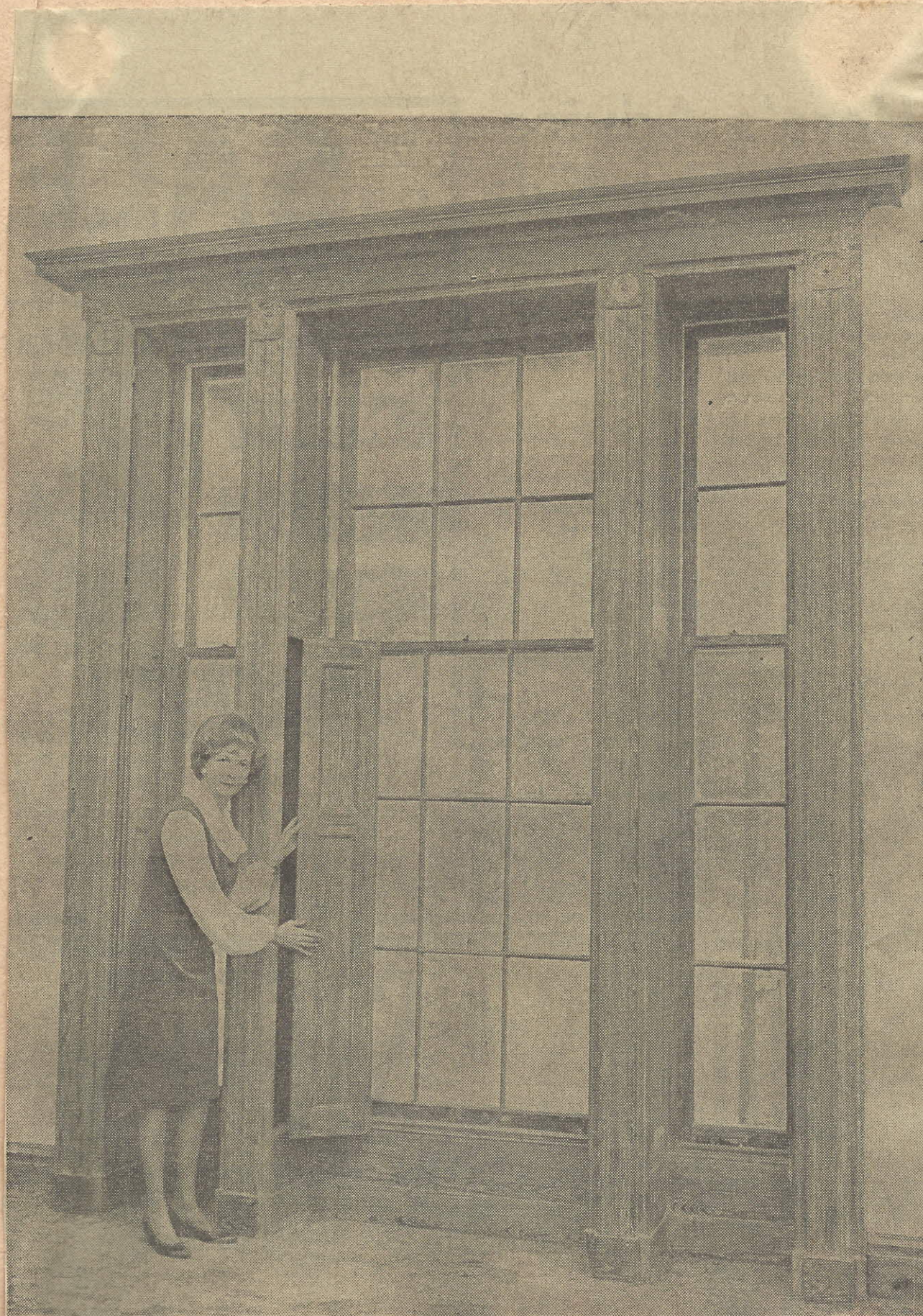
MRS. JAMES F. DREHER, president of the Historic Columbia Foundation, folds back one of the inside-panelled shutters on a window of the historic Ainsley Hall Mansion which the foundation is reconstructing. These three-part Venetian windows
