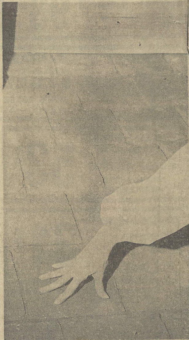
A CLOSE VIEW of the nine-inch tile brick pavers covering the ground floor of Ainsley Hall Mansion shows bricks laid without mortar in the joints. Sand has been swept between the cracks in 1820 fashion.
