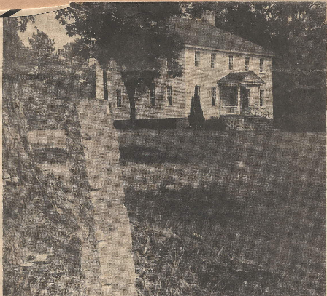
ACADEMY BOARDING HOUSE —Students attending Feasterville Academy were housed and fed in this handsome ante-bellum house which stands near the Academy. Well preserved through the years by the Mobley, Feaster and Coleman clans and other interested parties, the structure is a constant reminder of the determination man has had through the years to secure an education. Once a place buzzing with activity as well-to-do young men and women went about the task of securing an education, the remains of Feasterville Academy are somber except for the occasional chirp of a bird or the whisper of a breeze through the tall oaks which encircle the site.
