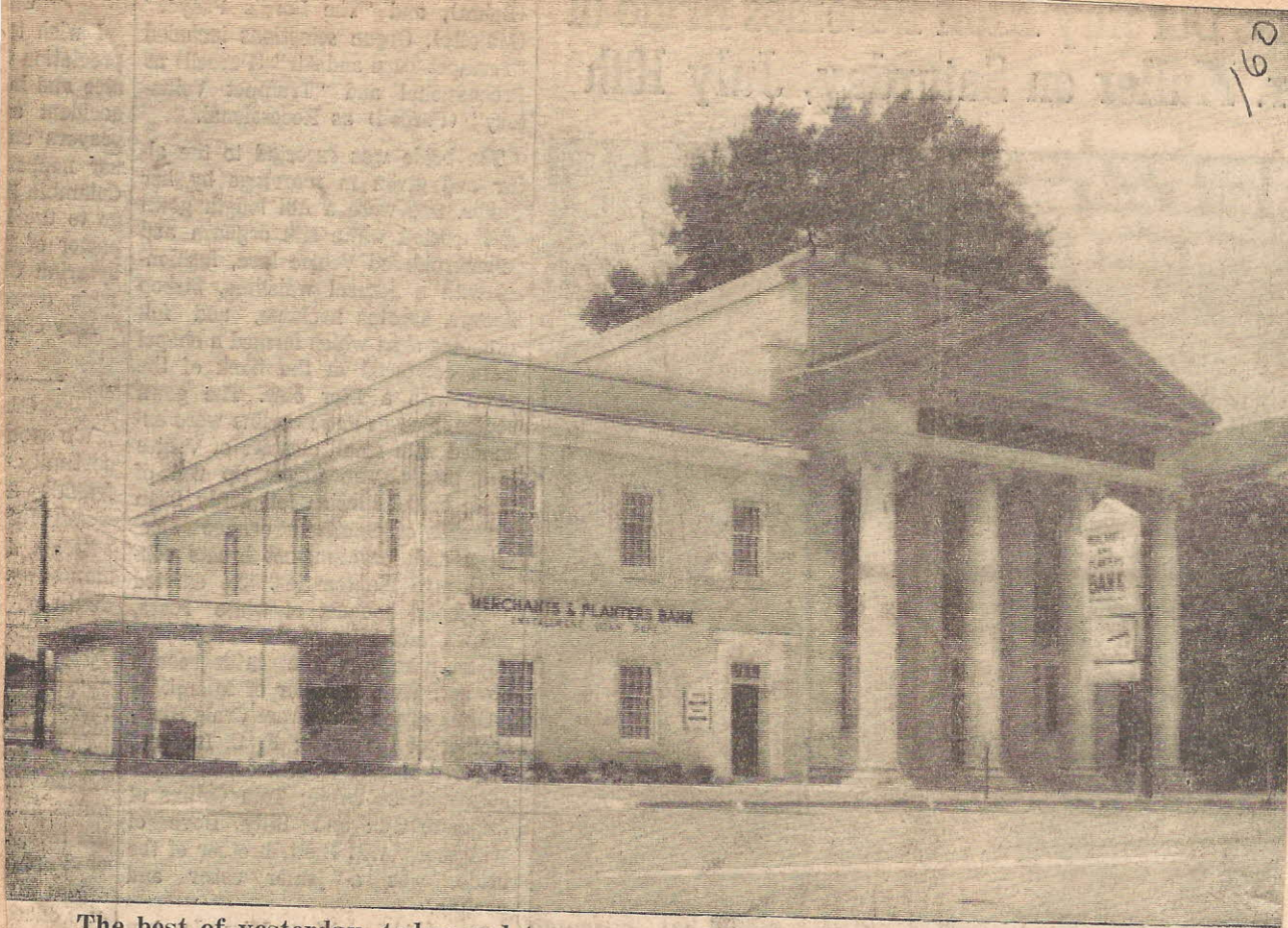
The best of yesterday, today and tomorrow are blended in the renovation and redecoration of this Winnsboro landmark.
