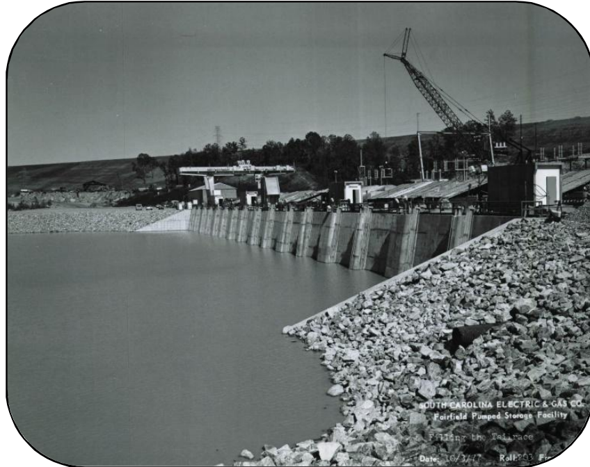
Filling of Fairfield Tailrace (1977)
