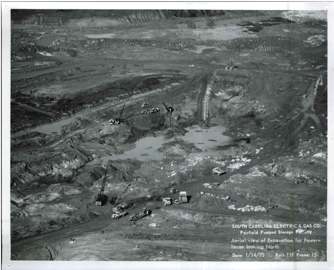
Excavation for Fairfield Pumped Storage
