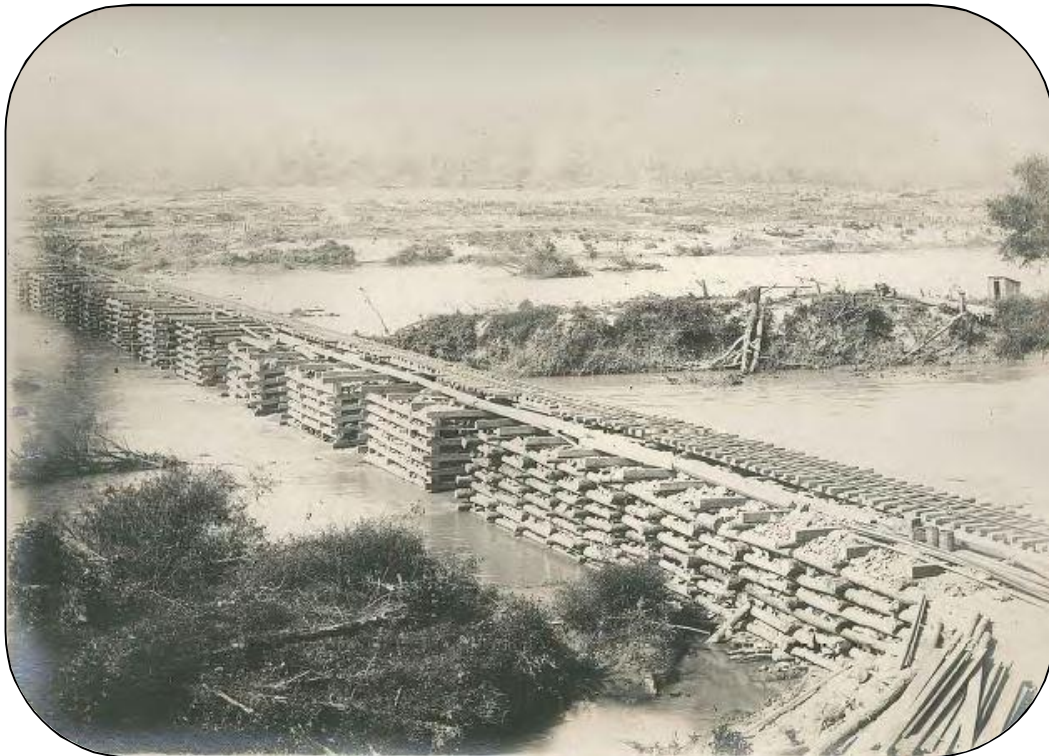
Coffer Dams used during the construction of the Parr Dam (1913)
