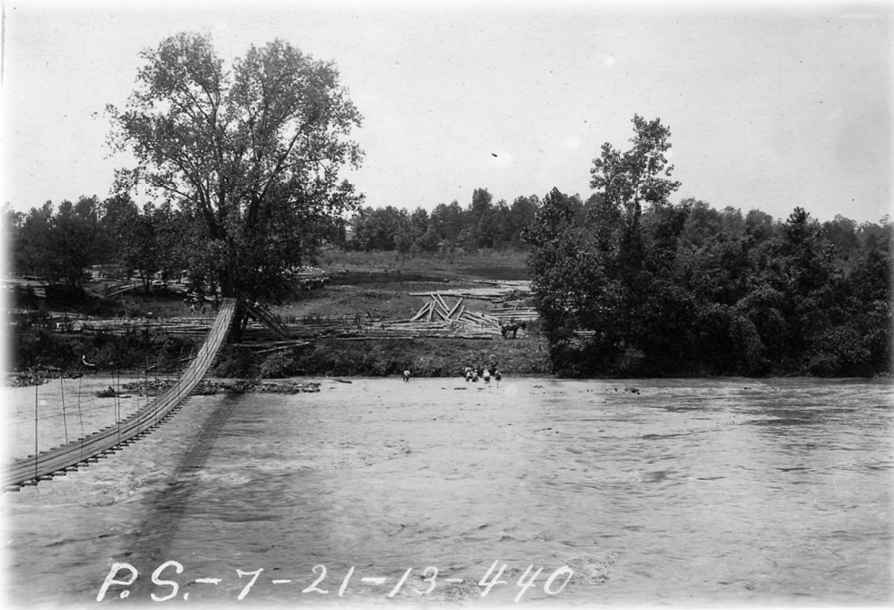
Bridge across Broad River during Parr Shoals Construction
