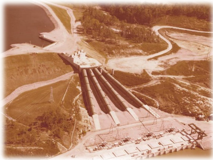
Fairfield Pumped Storage Facility after construction
