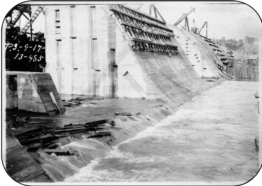
Parr Dam during Construction (1913)
