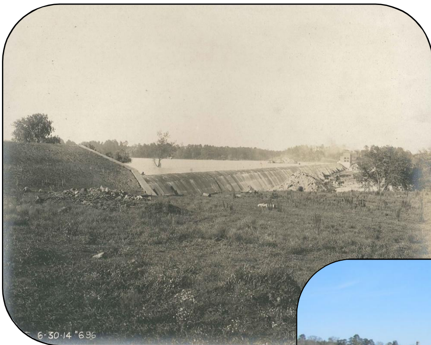
Parr Dam and Powerhouse (1914)
