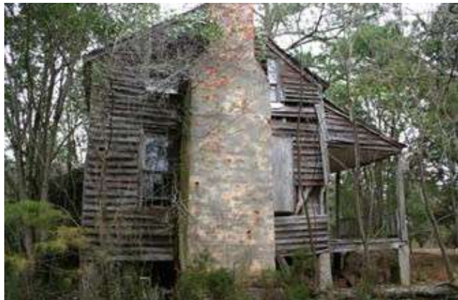
West end on left (Furman barracks). East end below shows clapboarding over log and deteriorated rear shed room and kitchen wall in far right.
