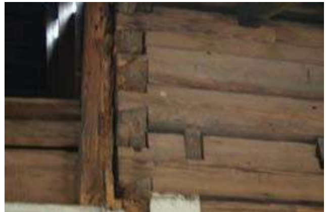
Detail of log notching on front of Hawthorne house visible under collapsed front porch
