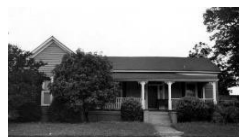
Charlotte & South Carolina RR House 1
