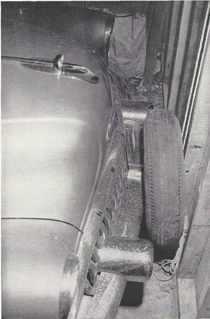
NAILING an old tire at back of garage enables driver to pull in closer. This, of course, allows more room for lawn mowers, baby carriages, bicycles, garden hose, tools borrowed from neighbors, etc.
